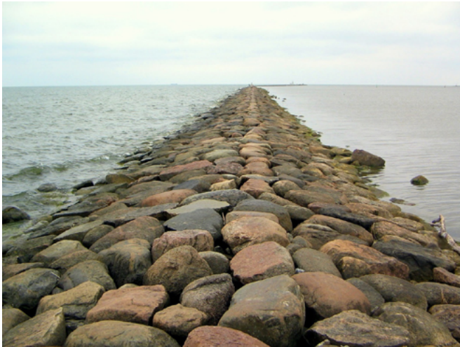
Breakwater. Source: Andrey Korchagin / Flickr
